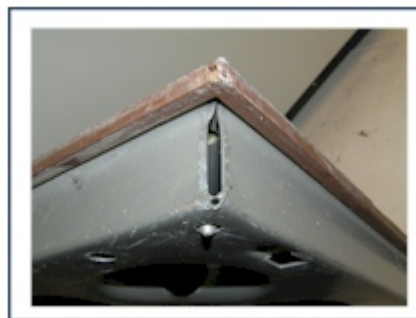
4. CORNER OF FLOOR PANEL
